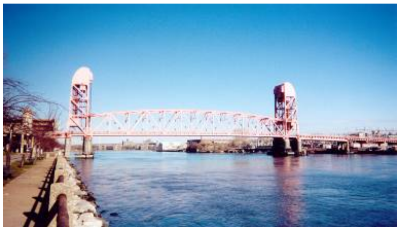
Fig. 1. Roosevelt Island Vertical Lift Bridge
